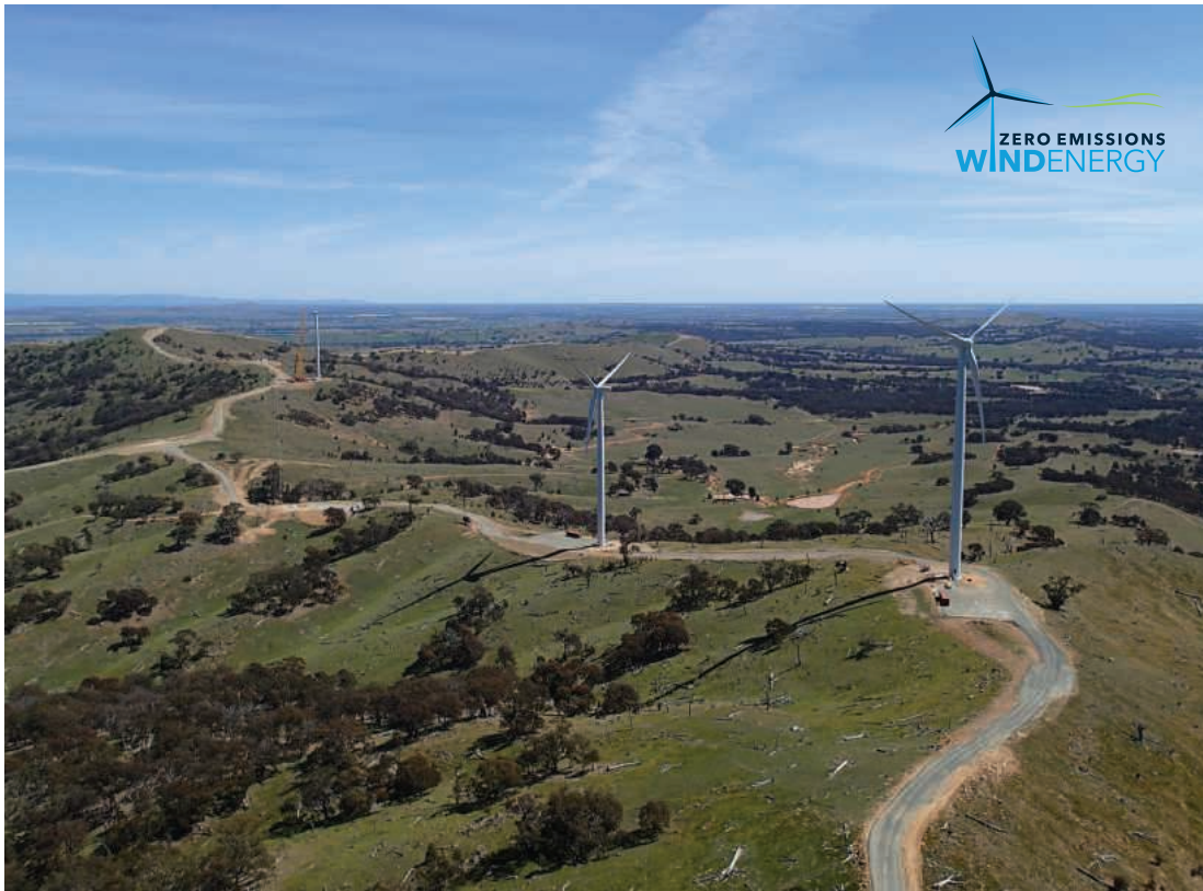
All Council's facilities – including libraries, streetlights, pools, gyms and town halls – are powered by 100% renewable energy from Crowlands Windfarm (pictured).
