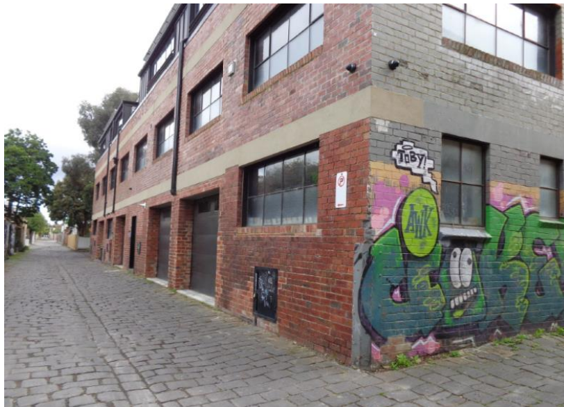
FIGURE 5: WAREHOUSE CONVERSIONS TO THE WEST OF REECE BRUNSWICK
