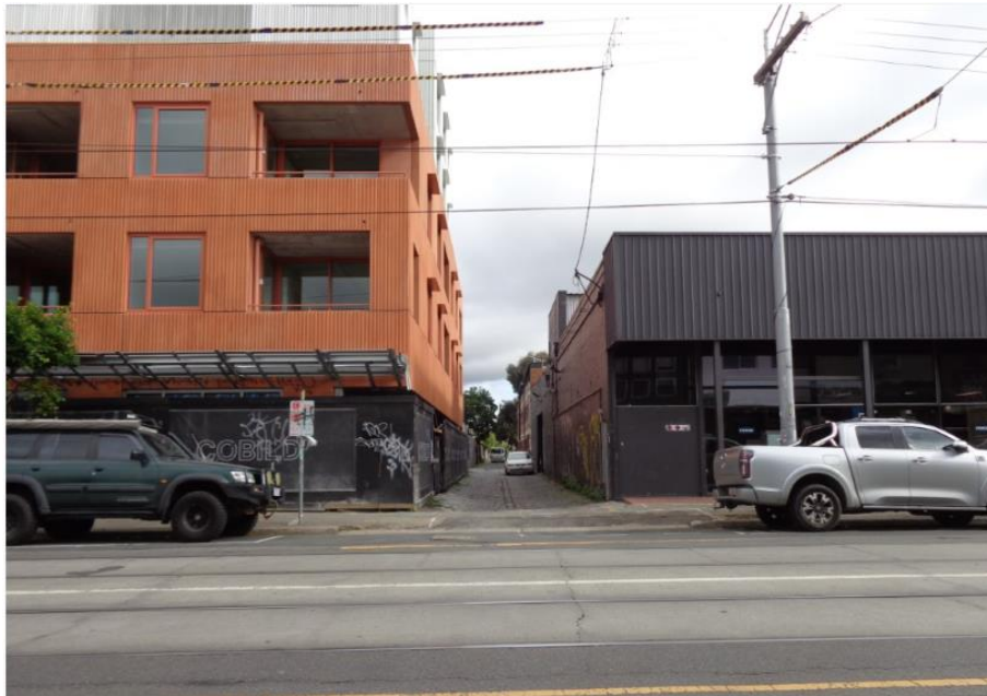
FIGURE 3: NEW APARTMENT BUILDING STILL UNDER CONSTRUCTION
