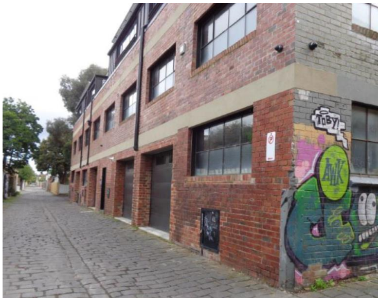
Figure 3: ‘No Parking Sign’ (with left-pointing arrow), Cocoa Jackson Lane, north side immediately west of Christopher Lane.
