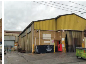
View 4 - Elm Grove facing south across to proposed apartment building site (former laundry drop forge factory)
