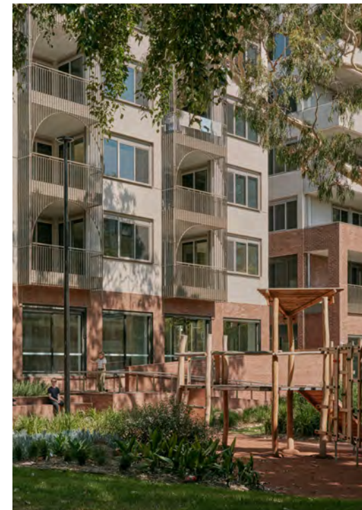
North Richmond Social Housing by Kerstin Thompson Architects and Hayball. Photo by Leo Showell.
