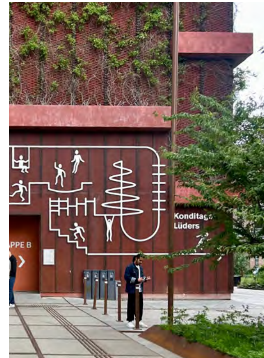
Multi-deck carpark in Copenhagen, Park 'n' Play by JAJA Architects. Photo by Katherine Sundermann.
