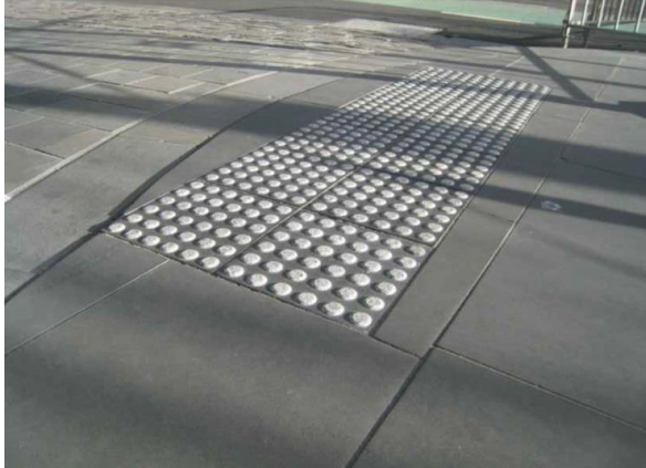
Granite studs within bluestone base
