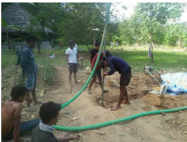
Installing water bore at Kadalak Dame Garden
