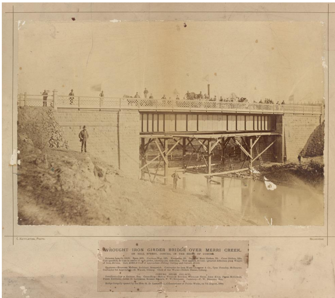
Wrought iron lattice girder bridge over Merri Creek, Charles Nettleton 1826-1902, photographer. View shows men, horses, and steam engine on a bridge, with three men on the banks beside the river. (Source: SLV, Accession no(s) H85.153/2)
