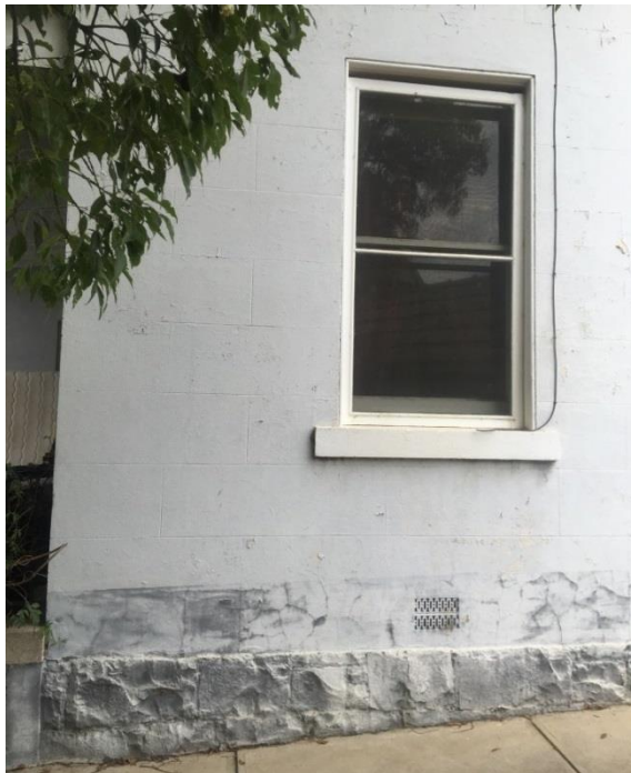
Figure 12: Fenestration, bluestone foundations and cast-iron vent pattern are evidence of the Victorian origins of the existing dwelling on the subject site (source: Context 2016)
