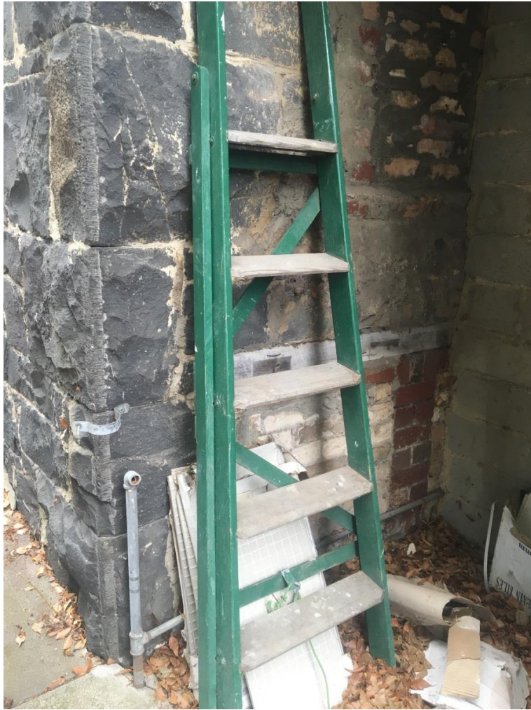
Figure 16: Brick infill to openings on east elevation (source: Context 2016)
