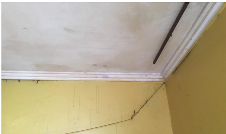
Figure 19: Bluestone building has c.1930s masonite lining and Art Deco cornicing (source: Context 2016)
