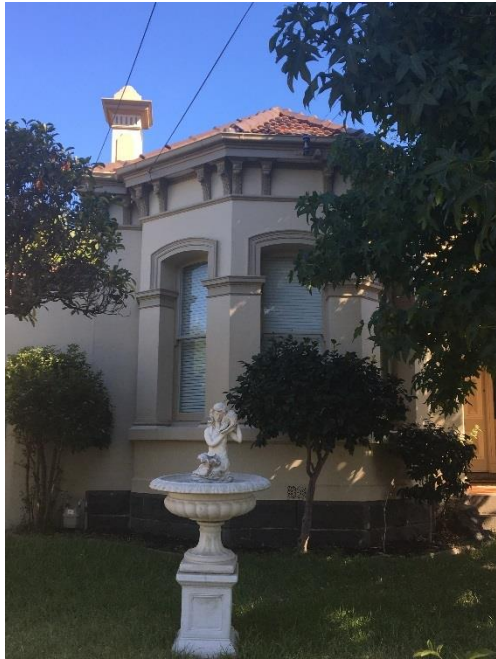
26 Walsh Street Coburg – detail of canted bay and acanthus leaf brackets (Source: Context Pty Ltd)
