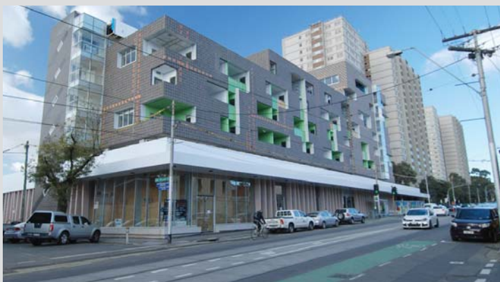
2.4.1 Solid balustrade for balconies reduces the noise transmitted into the apartment from busy road
