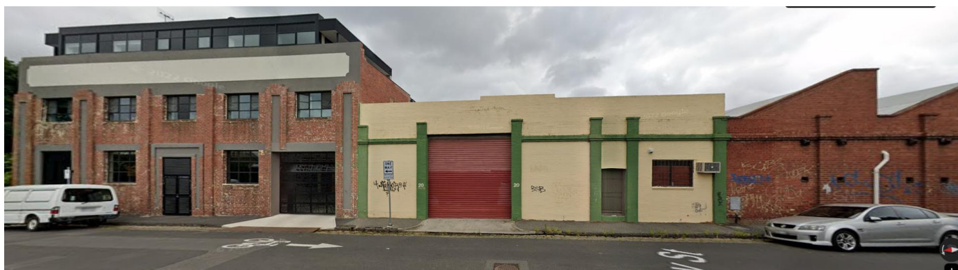
Figure 5 - The former factory's building styles along the Gray Street frontage
