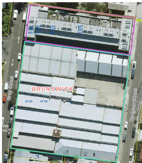
Figure 4 - Aerial view of site with the northern and southern parcels outlined in purple and green respectively
