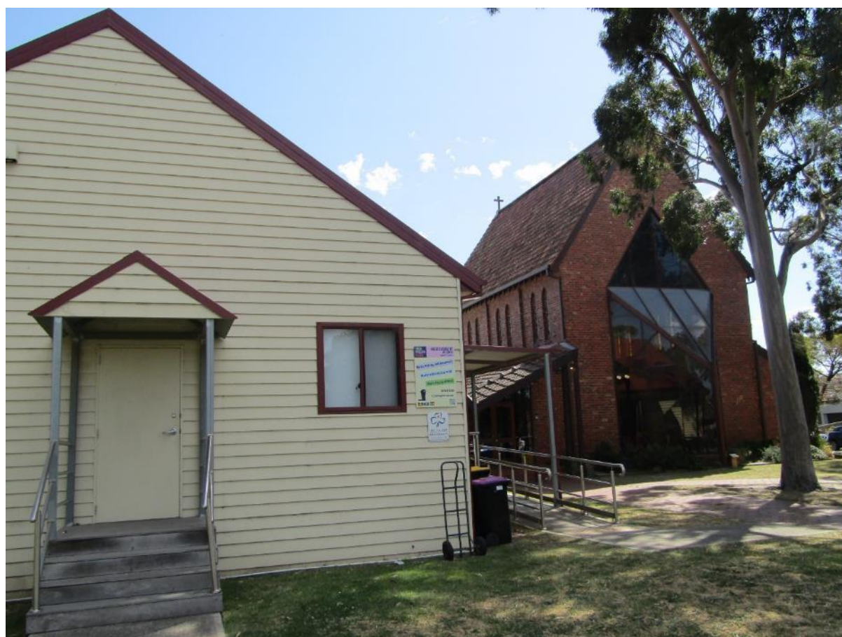
Figure 15. View of east elevation of St Linus Church and the hall.
