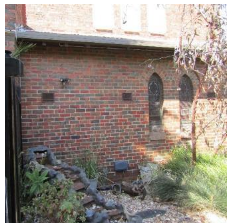
Figure 20. View of lower west elevation.
