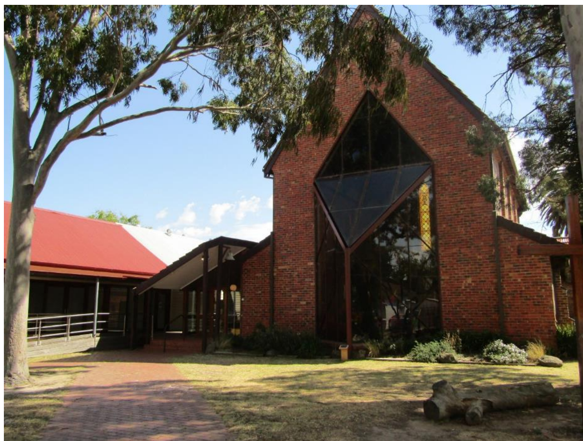
Figure 16. View of east elevation of St Linus Church, showing later addition of glazed window.
