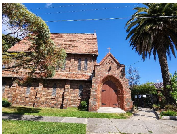
Figure 17. View of north elevation showing buttressed piers and stained-glass windows, and Canary Island Date Palm.
