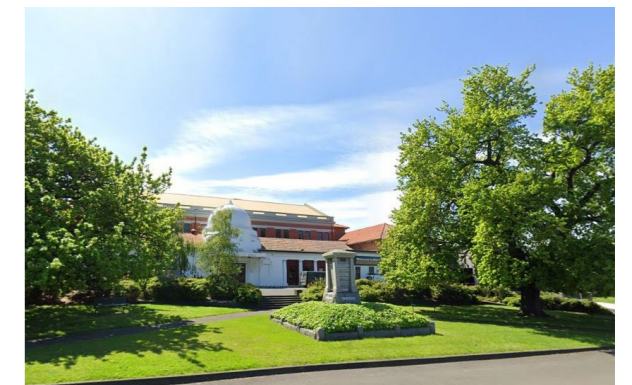
Figure 26. Municipal Office Forecourt
