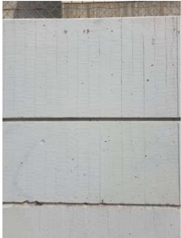
Detail of off-form concrete boundary wall.
