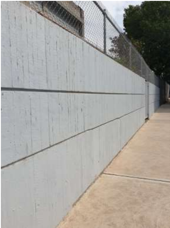
Detail of off-form concrete boundary wall.
