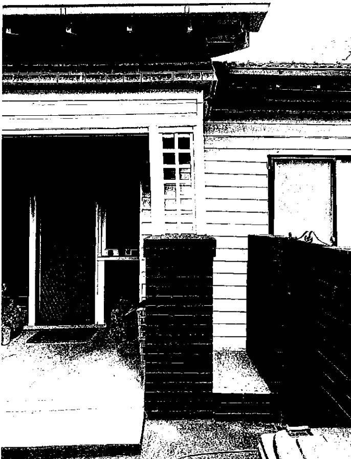
Figure 8 - Supporting pillar near entry is leaning severely
