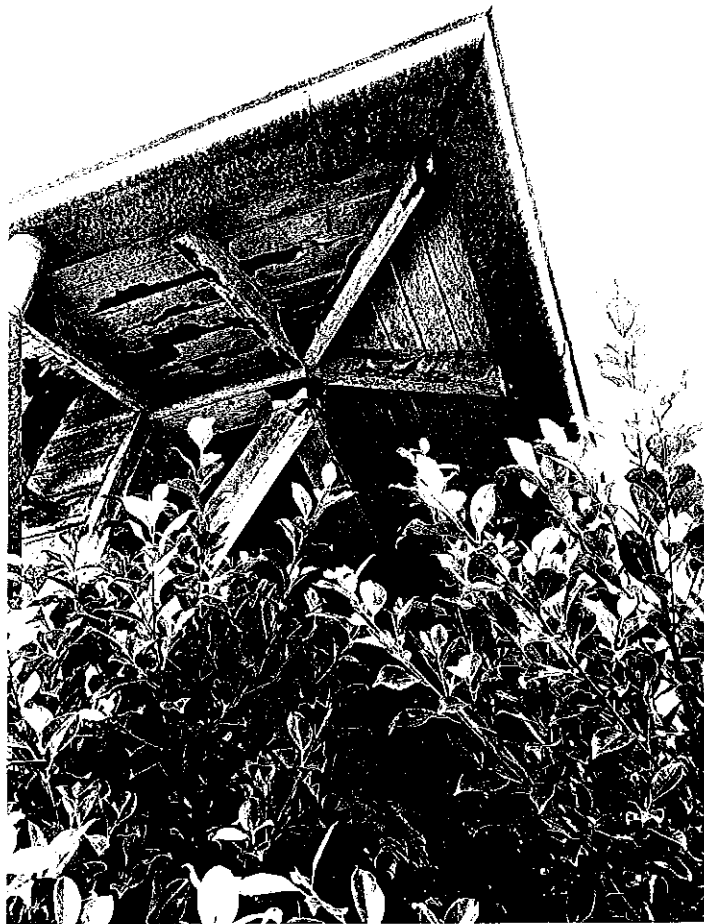
Figure 9 - Under side of eaves decaying
