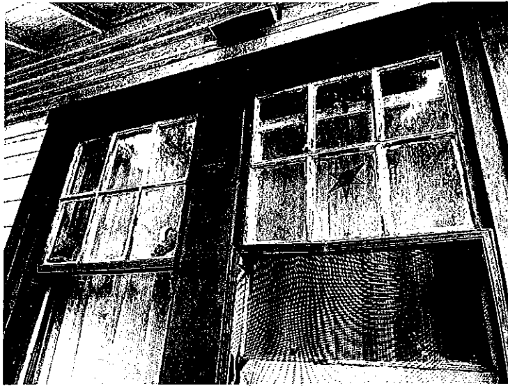
Figure 5 - All original window frames are rotten
