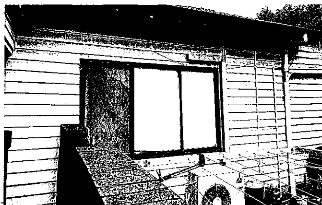
Figure 1 - View of non-original window on eastern elevation
