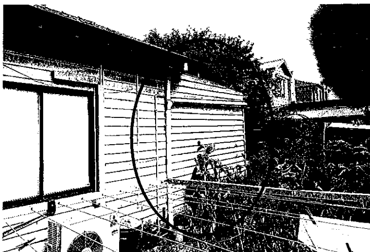
Figure 3 - Lean-to visible at rear of dwelling
