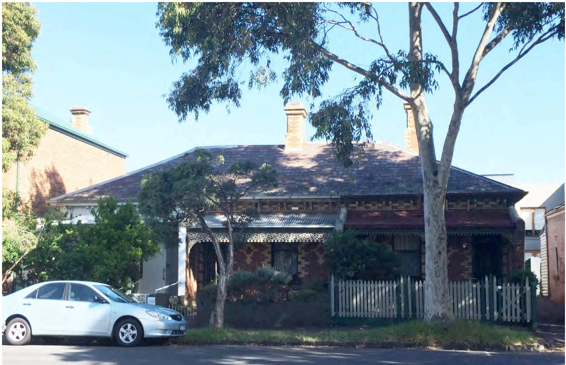
Terrace, 206-210 Barkly Street, Brunswick. No. 210 is the house on the right.
