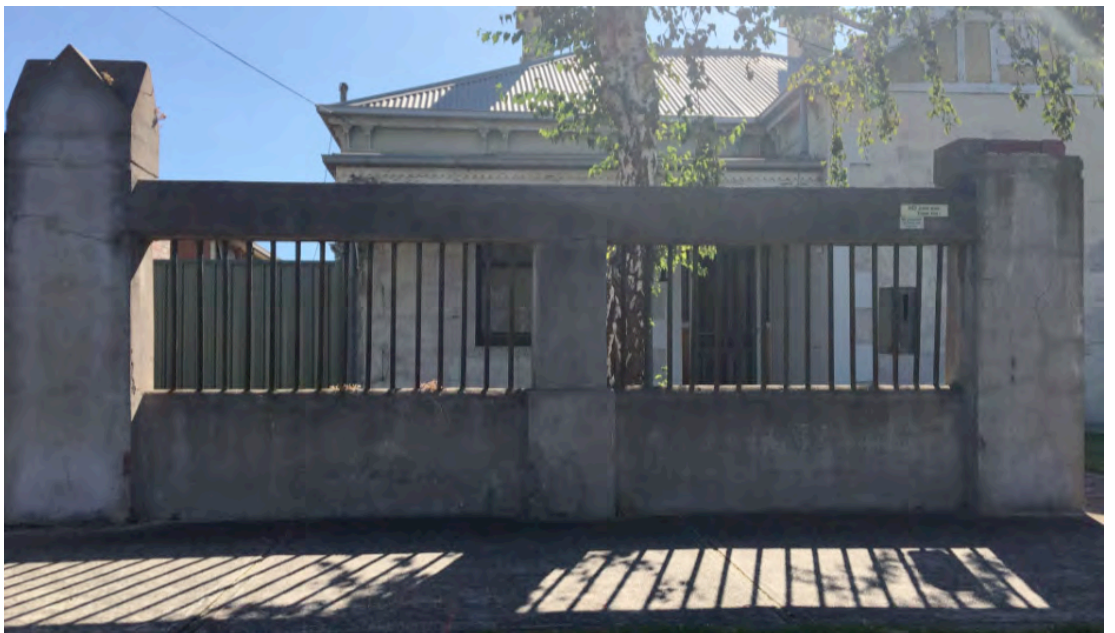
House and front fence, 1 South Daly Street, Brunswick West
