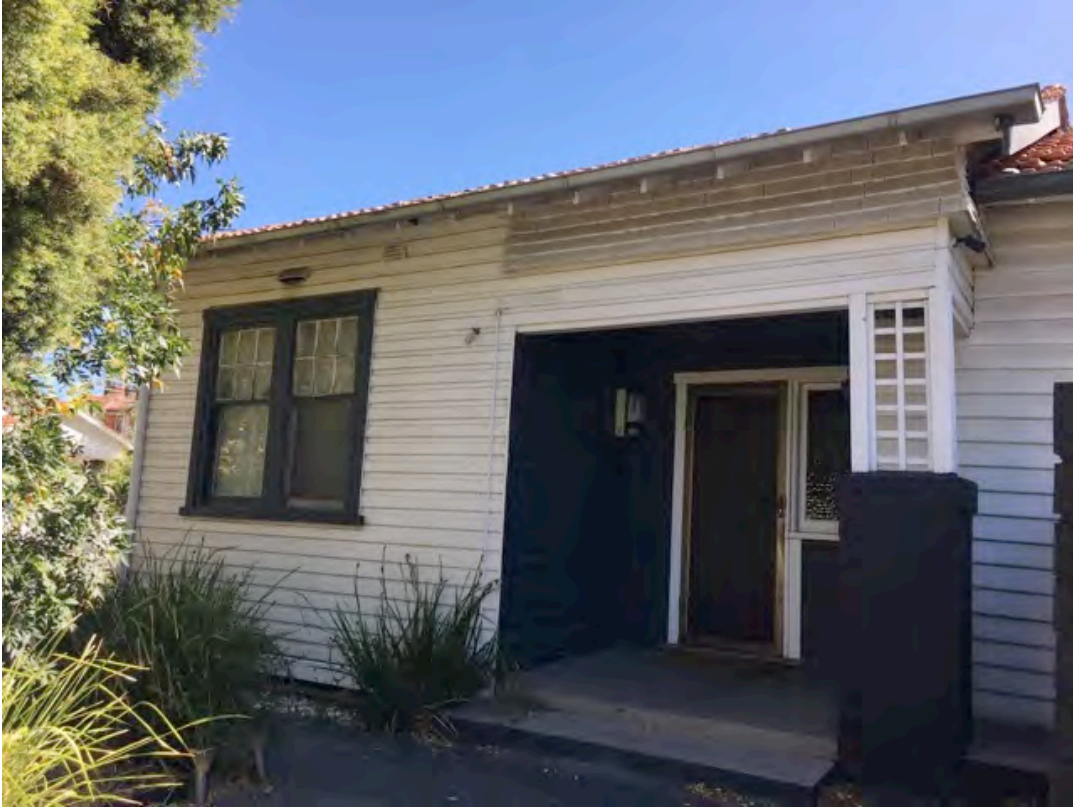
House, 183 Stewart Street, Brunswick East
