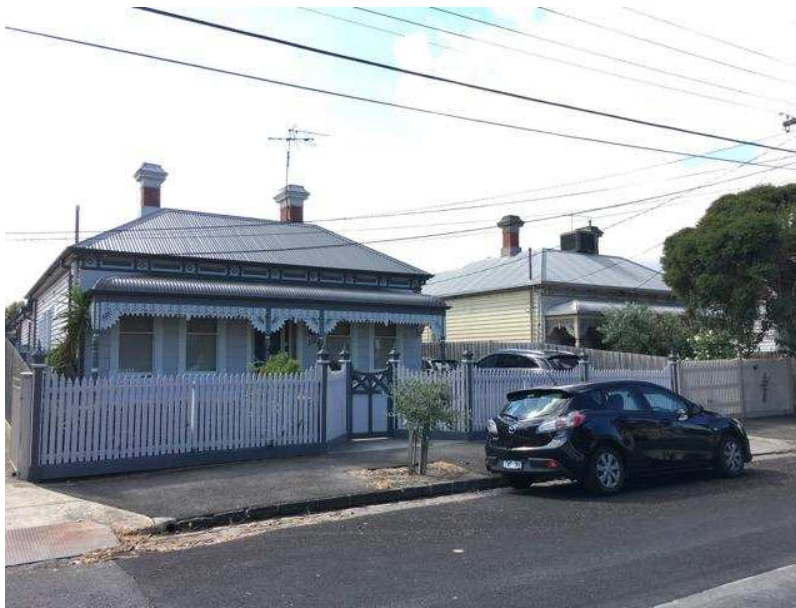
Tinning Street Precinct - nos. 110 and 112
