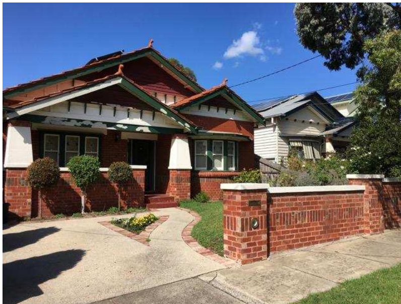
Meaker Avenue Precinct
