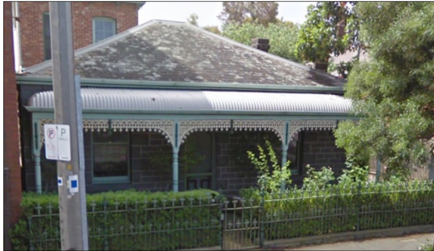
Figure 25 1860s bluestone cottage, 193 Weston Street, Brunswick (HO195).
