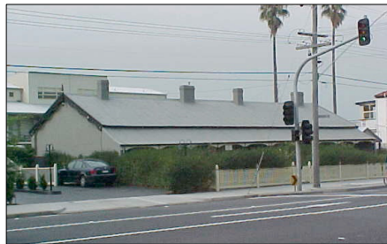
Figure 9 (left) 181-189 Brunswick Road, Brunswick. Prefabricated iron houses, constructed c1854 (VHD H1151).
