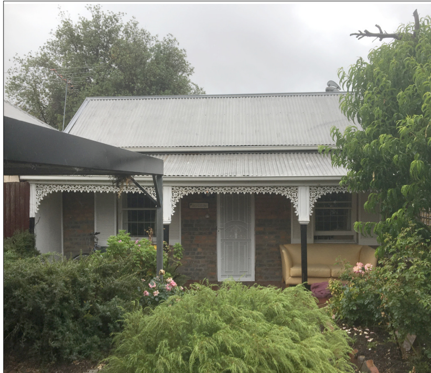
Figure 3 The front elevation. Note how the posts above the capitals have been extended sideways in order to make the cast aluminium frieze fit – this seems to be a modern detail arising from the use of a modern frieze.
