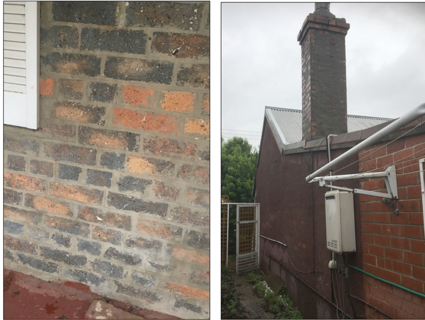
Figure 6 (left) Detail of the front façade showing bricks of varying colour (many overfired clinkers) and modern cement rich pointing.
