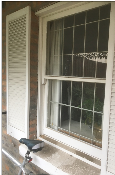
Figure 4 (left) Detail of the front façade showing non-original window frame and shutters.
