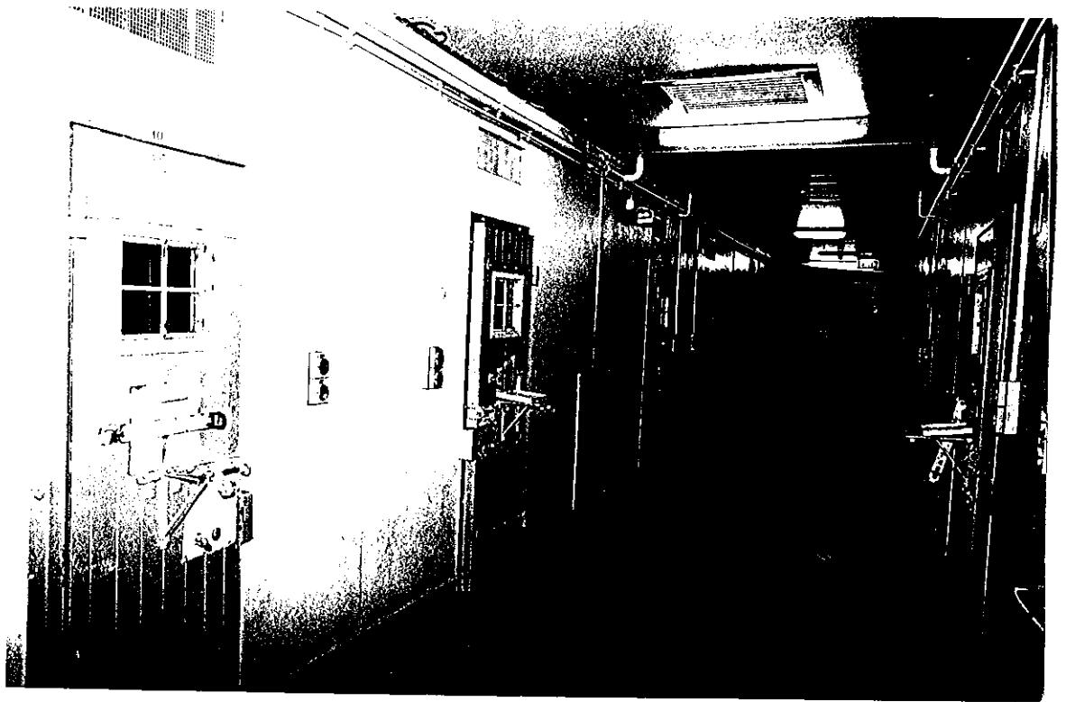
Figure 118 Interior of the 1959 cell block, showing the rehung original doors in the north section of the west wing
