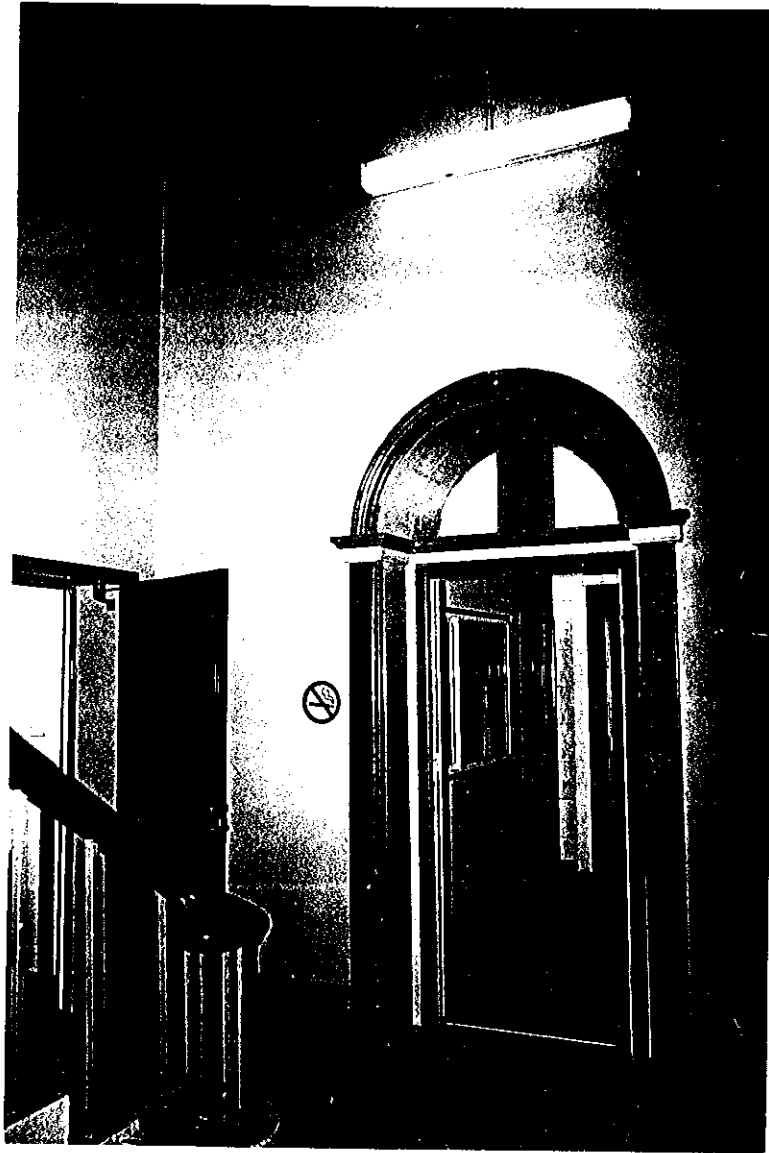
Figure 57 Doorway in rear wall of entrance vestibule, showing original joinery
