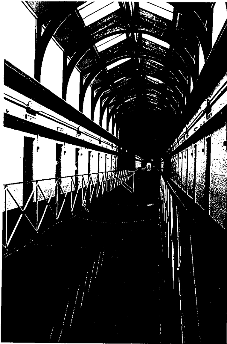
Figure 125 Galleried corridor looking west, showing the iron galleries and the arched timber roof trusses
