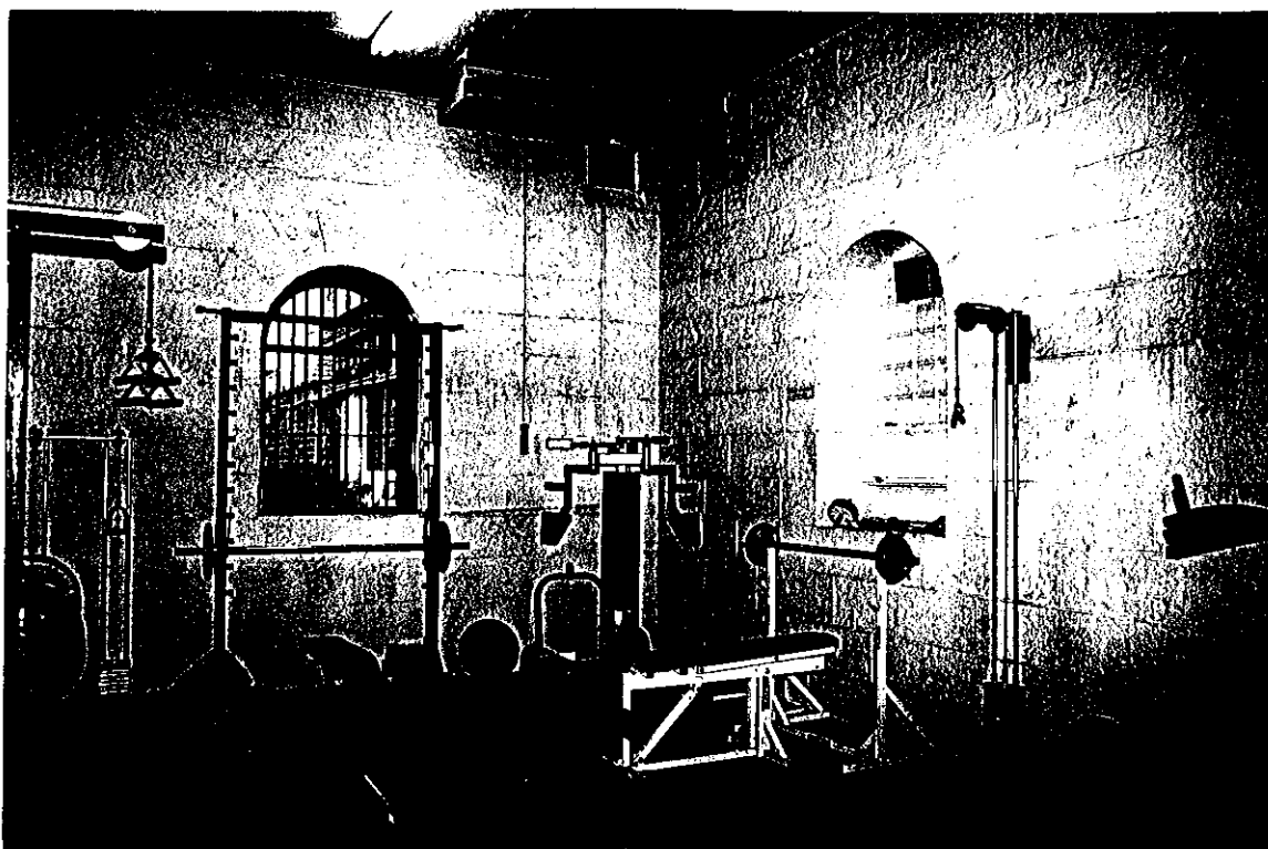
Figure 56 Former ward at south-west corner of ground floor, showing painted bluestone walls and concrete ceiling
