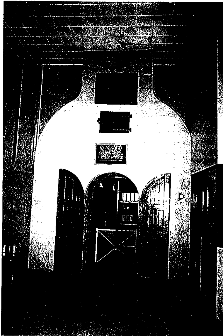
Figure 70 Ventilation stack in first floor chapel, showing twin doors to furnace and ash chamber
