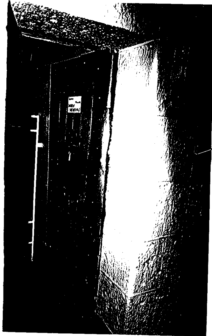
Figure 75 Cell door in the west wing, showing framed and boarded construction, original hinge pivots and strap reinforcement and later steel hatch
