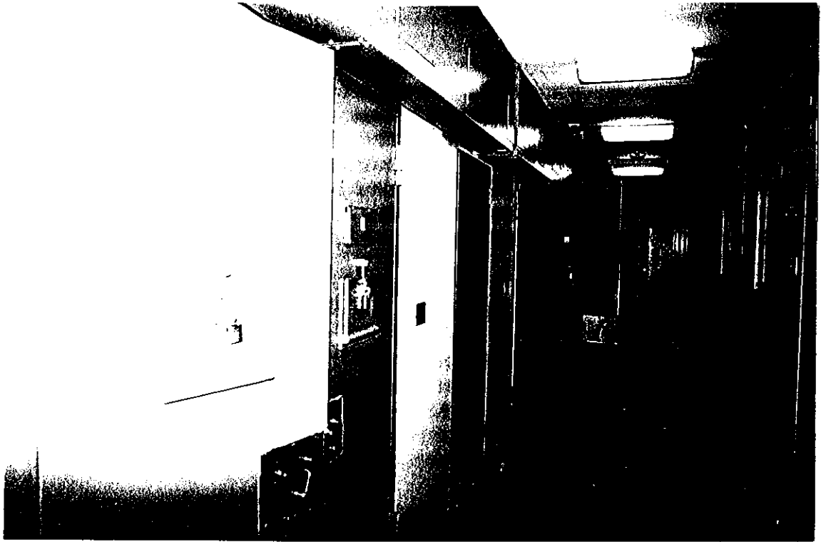
Figure 164 View of the corridor in front of the cells, showing the replacement hinged cell doors and the casings to the original pneumatic door operating mechanisms
