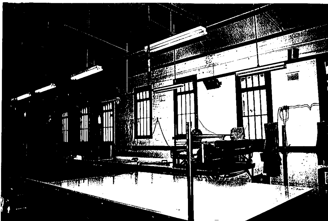
Figure 92 Interior of Tailors' Shop, showing the original windows. The higher windows in the centre indicate the location of the original overseer's room which originally divided the space into two workshops
