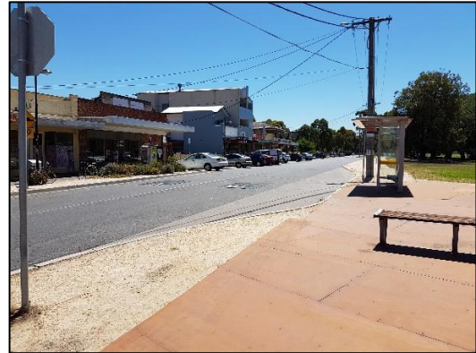
Figure A.26: Merlynston Station Activity Centre
