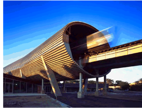
QB17 McCormick Tribune Campus Centre, Chicago, USA Noise-absorbing steel tube wrapped around metro to protect The McCormick Tribune Campus building
