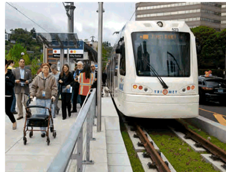
QB4 MAX Orange Line, Portland, USA Vegetated trackway for stormwater benefits
