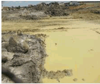
Image: Poor site management results in sediment laden stormwater making its way into creeks.
