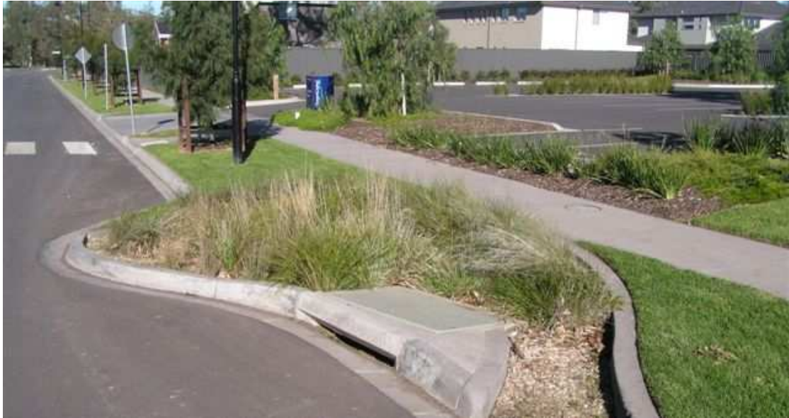
Photos 5 and 6 BRS inserts to road pavement/footpath verge at Mernda Villages. In the photo above bioretention swales are also integrated into the carpark buffer spaces within the pavement area.
