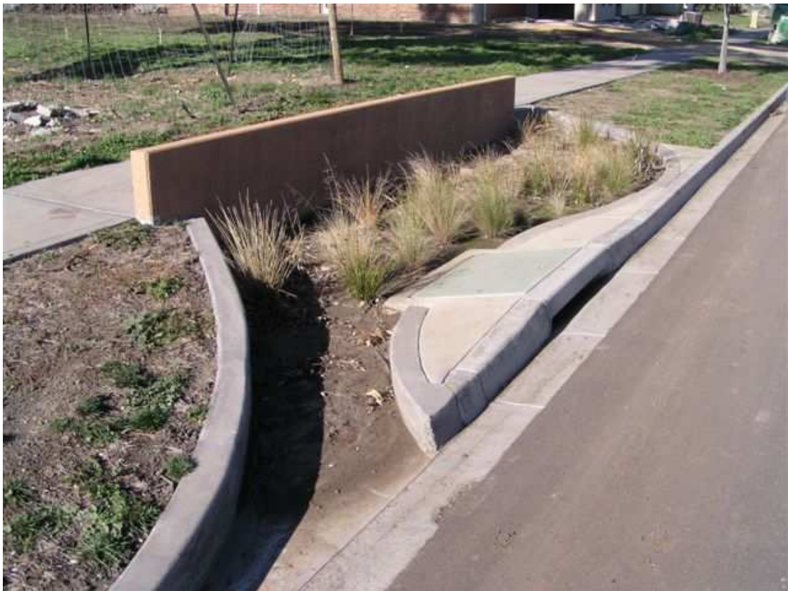
Photos 5 and 6 BRS inserts to road pavement/footpath verge at Mernda Villages. In the photo above bioretention swales are also integrated into the carpark buffer spaces within the pavement area.
