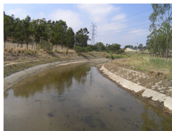
CONCRETE LINED CHANNEL SECTION OF EDGAR'S CREEK
