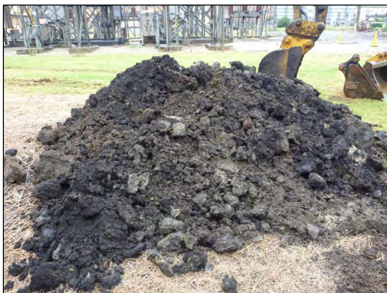
PHOTOGRAPH 2 – TEST PIT 1 SPOIL
