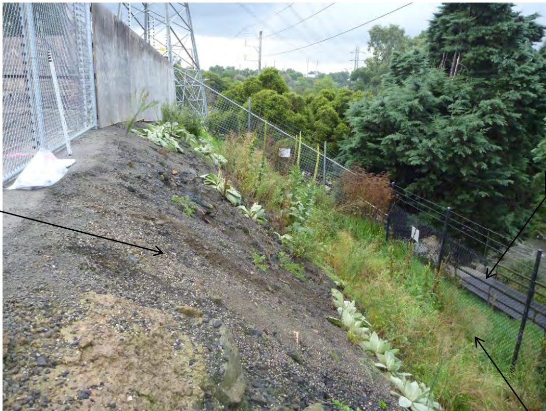
PHOTOGRAPH 3 - FILL BATTER (SECTION C-C')
