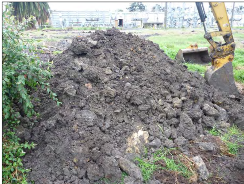
PHOTOGRAPH 4 – TEST PIT 2 SPOIL
