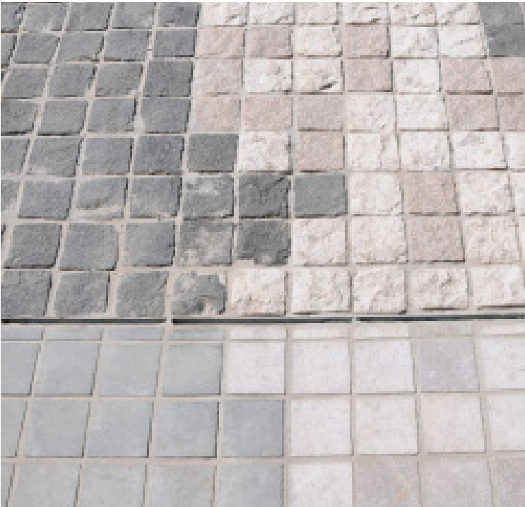
Combining natural split and sawn cut finishes - smooth finish for ease of manouvering shopping trolleys over paving and for mobility and access requirements.
