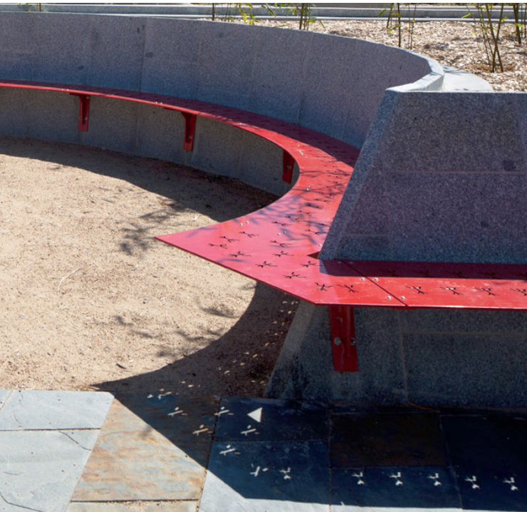
Feature seating mounted on planter walls
