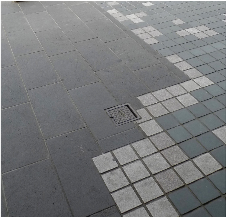
Combining bluestone slabs & granite setts
