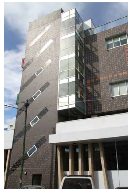
example of surface treatment of facade to provide detail and break down mass
