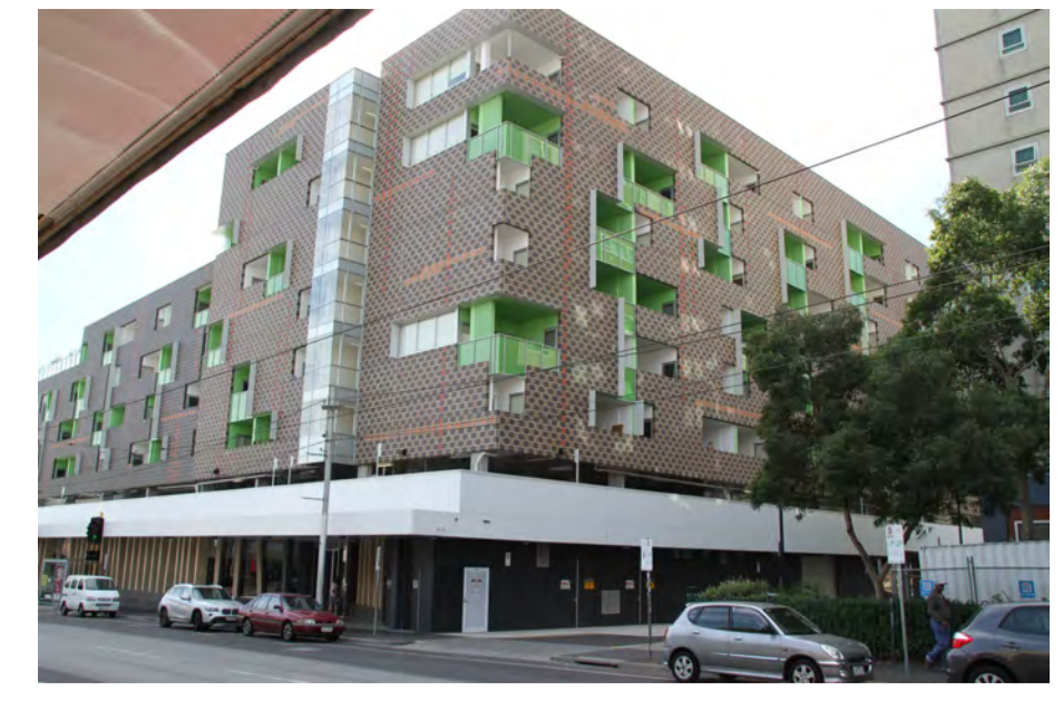
example of recesses / voids used to break down the mass of a facade colour has been implemented to the recesses to provide depth to the facade
