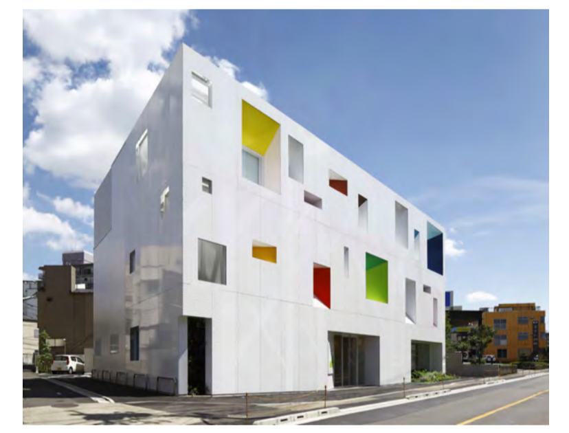
example of recesses / voids used to break down the mass of a facade
