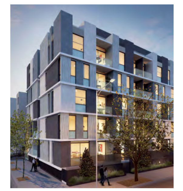
example of expressed floor slabs to provide an emphasis on horizontal planes on a facade to minimise bulk - also use of alternating colored panels assist in minimising bulk
