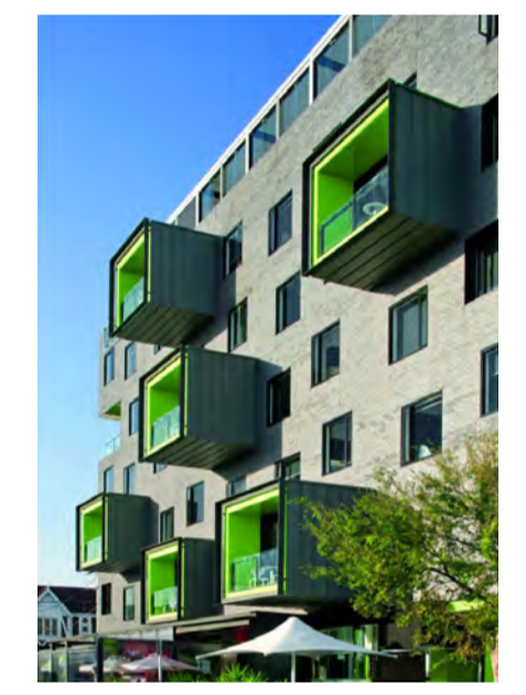
example of projecting elements with highlight colors to provide depth and focal points to a simple facade
