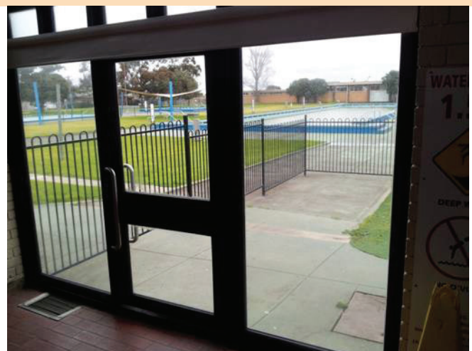
AFTER DOUBLE GLAZING
